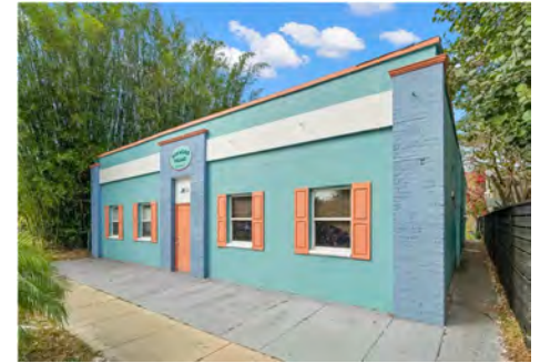
KENWOOD VILLAS 2409 4TH AVE N ST. PETERSBURG, FL
