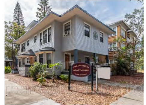
THE COLISEUM APTS 610 5TH AVE N ST. PETERSBURG FL
