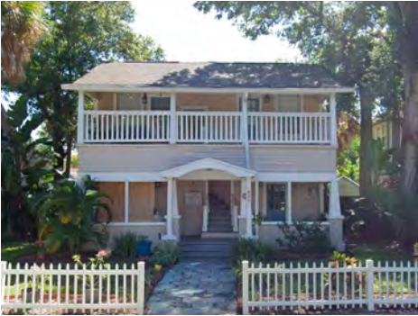
VILLA VERANDA 829 5TH ST. N ST. PETERSBURG, FL
