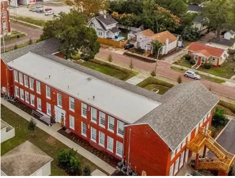
SCHOOL HOUSE APTS 1090 10TH ST. N ST. PETERSBURG, FL
